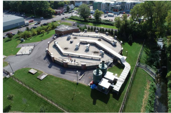
Lower Harbor Brook Storage Facility.
