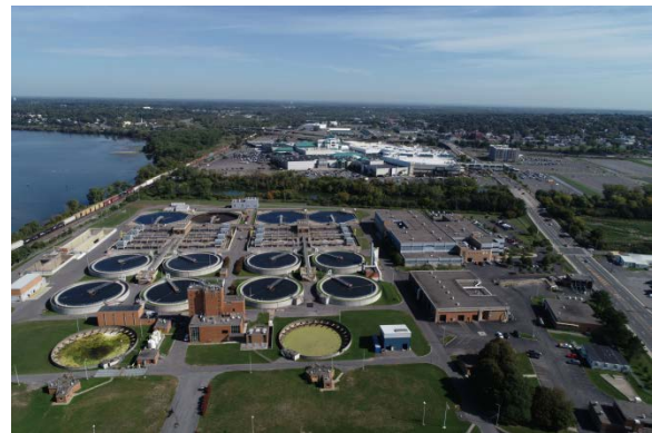
Aerial View of the Metropolitan Syracuse Wastewater Treatment Plant.
