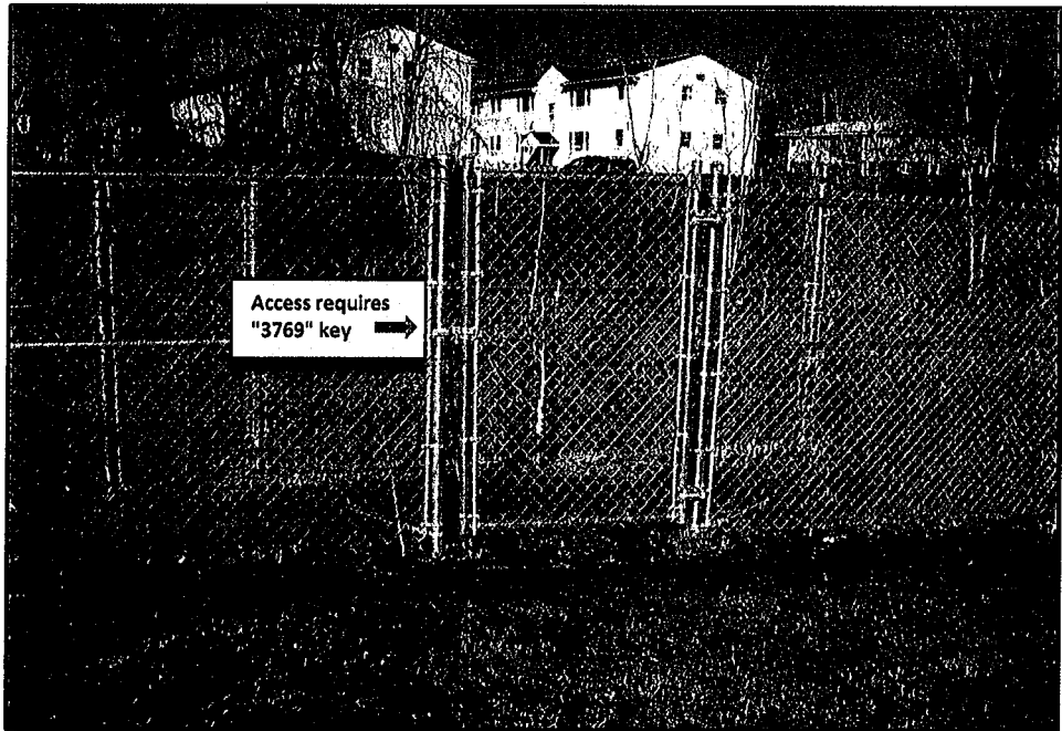
Midland RTF Outfall @ Creek
