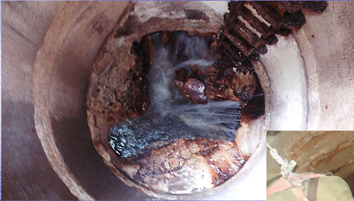
Leaking manhole before
