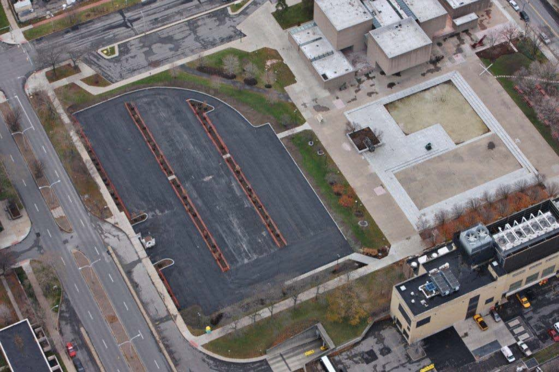
Base Course Asphalt Installed prior to winter shutdown
