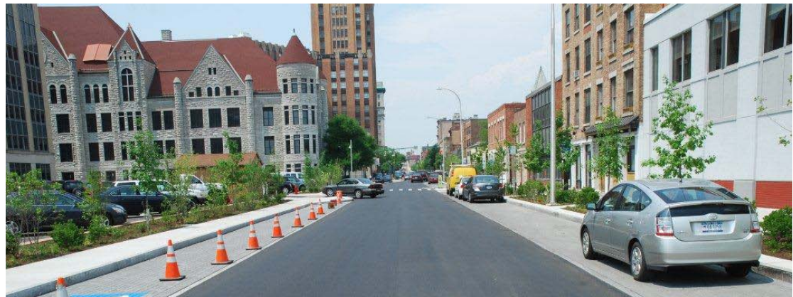
“Gateway Project” 300 Block of East Water Street, Completed 2011-12
