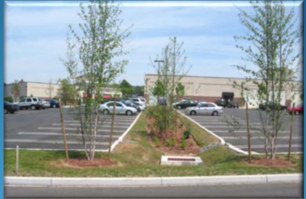
A typical parking lot bio-retention island
