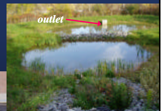
Stormwater Pond with controlled outlet
