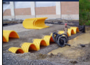
Stormwater Pond with controlled outlet
