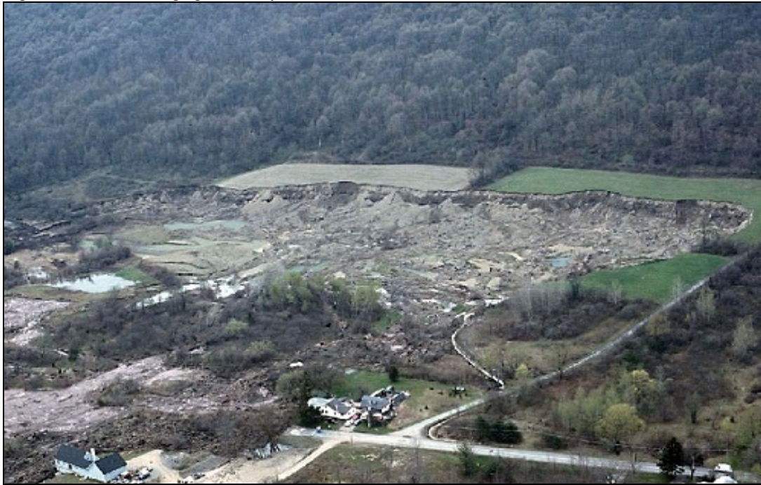
Figure 5.4.4-14. Photograph of Tully Farm Road Landslide
