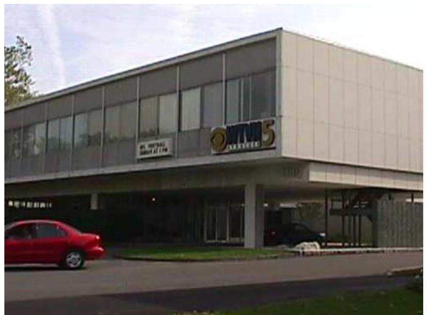
MODERN PLANNING: RECENT JAMES STREET BUILDINGS TAKE A FORM THAT POORLY DEFINES THE PUBLIC REALM AND DISCOURAGES PEDESTRIAN ACTIVITY.
