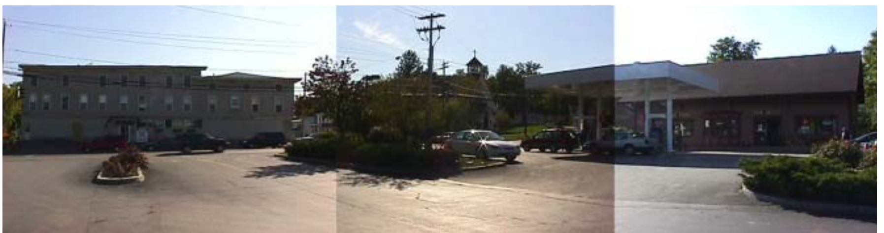
THE JAMESVILLE INTERSECTION, WITH ITS CORNER ERODED BY THE GAS STATION
