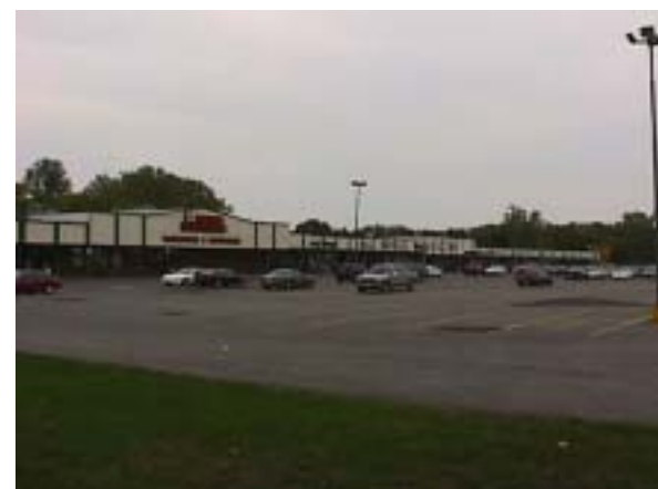
THE BAYBERRY PLAZA: POORLY PLANNED, BUT EXTREMELY USEFUL
