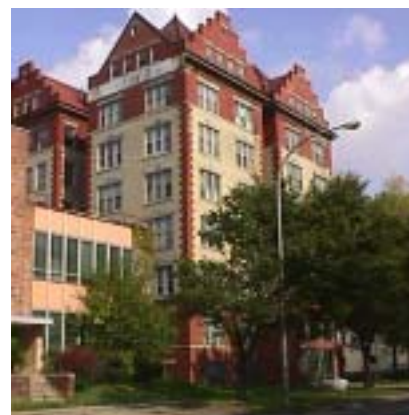
1. URBAN CORE: TALL APARTMENT BUILDINGS AND OFFICE SIT CLOSELY AGAINST A WIDE SIDEWALK FRONTING A HEAVILY-TRAFFICKED THOROUGHFARE. (JAMES STREET)
