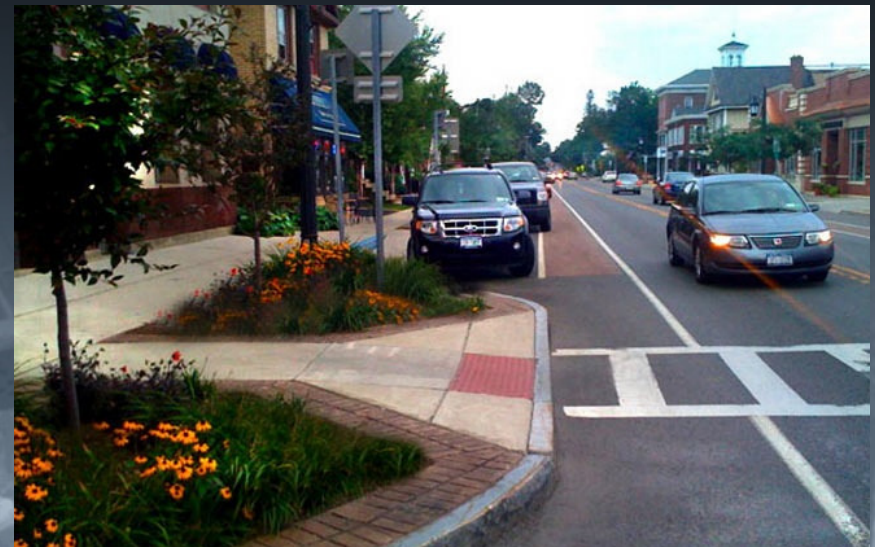
Intersection Curb Extensions
