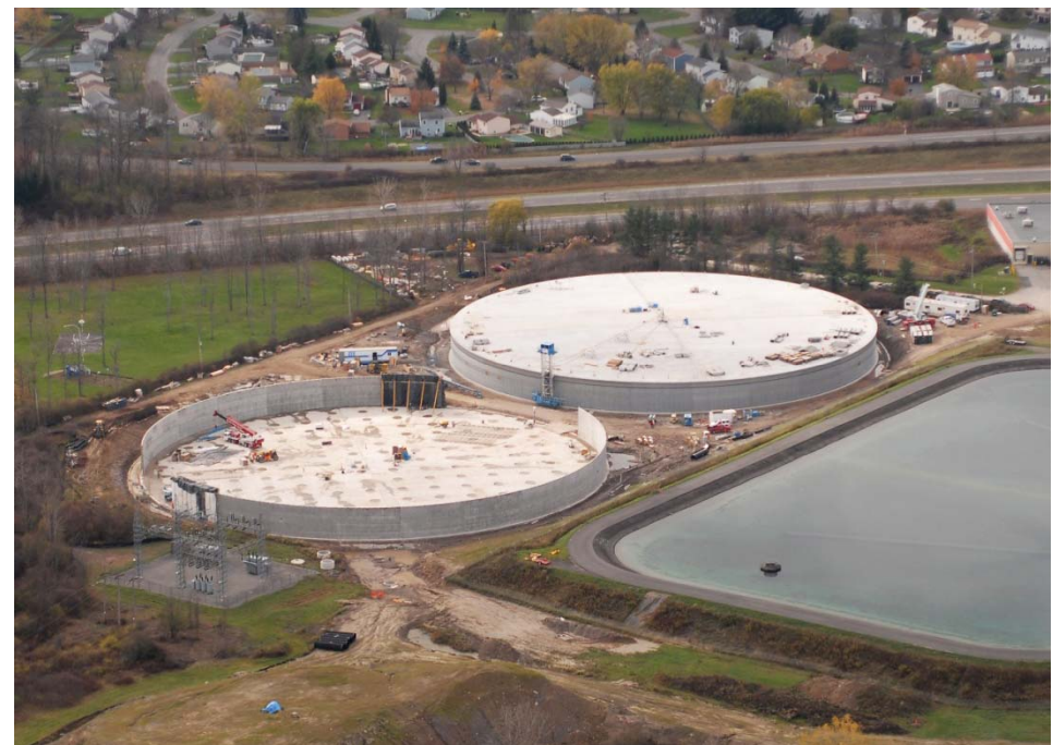
MWB Reservoir, Town of Clay
