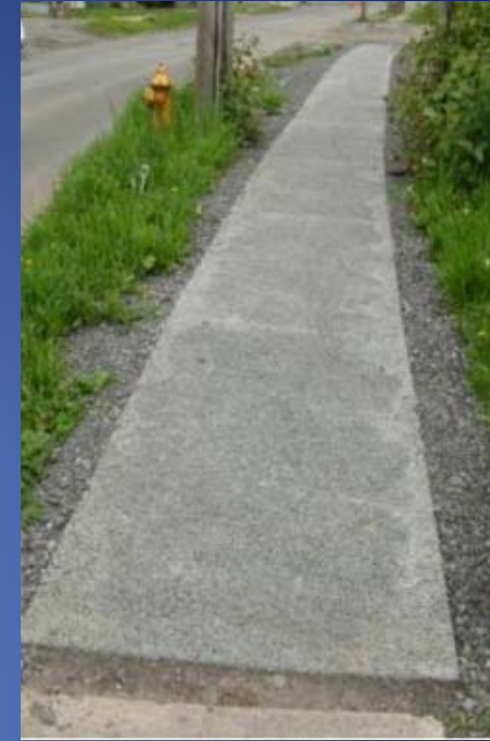
Grand Avenue Porous Pavement Sidewalk Test Segment OCWEP / Save the Rain
