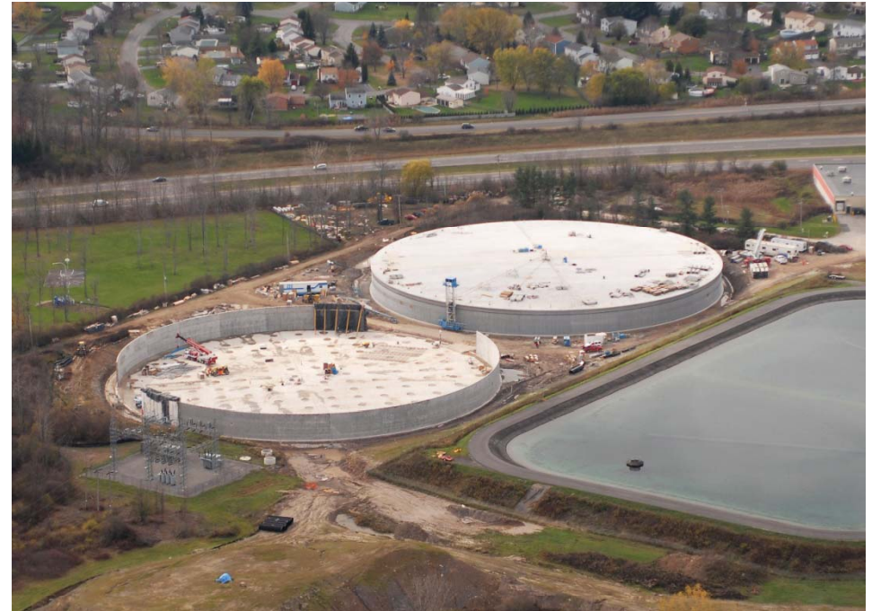
MWB Reservoir, Town of Clay
