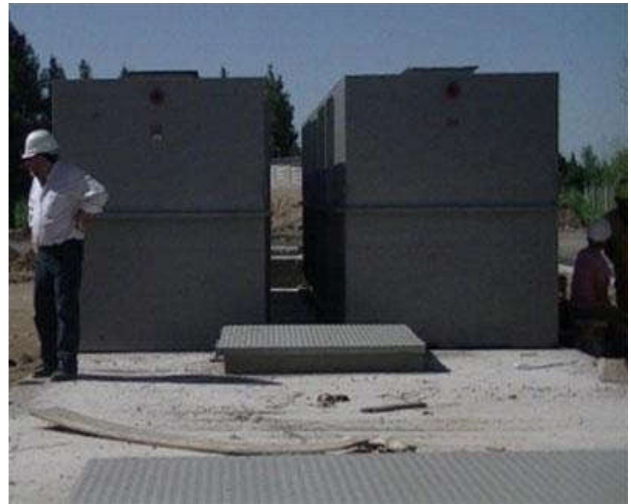
Sewer Package System
