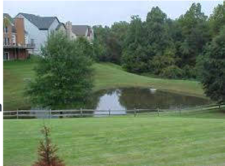
Stormwater Detention Pond
