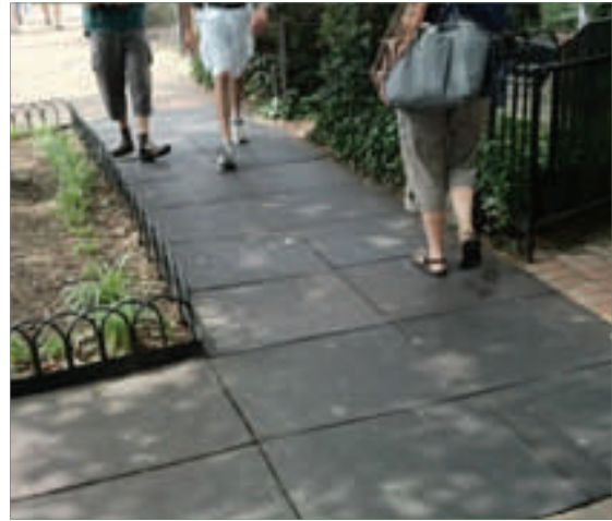
Rubberized sidewalk pavers. Photo credit: FHWA.
