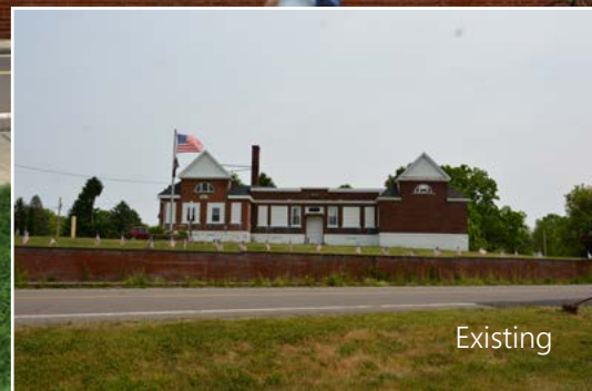
Proposed - Restoration of the original window openings in the American Legion celebrates the historical importance of the former community school.
