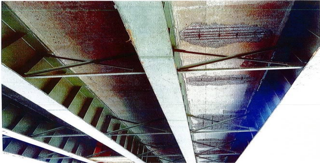
Emergency deck repair I-690
