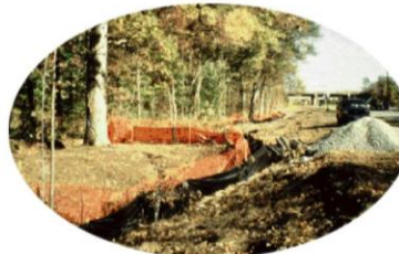
5. Erosion & Sediment Control
