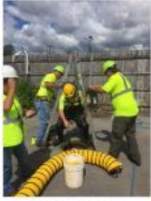
Ensuring safety in confined spaces.
