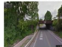
Bear Trap - Ley Creek N. Midler Culvert Rehabilitation
