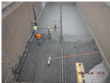
$25 million project to maintain and meet new SPDES compliance by April 2017.
