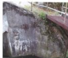
Harbor Brook Drainage District Culvert Rehabilitation
